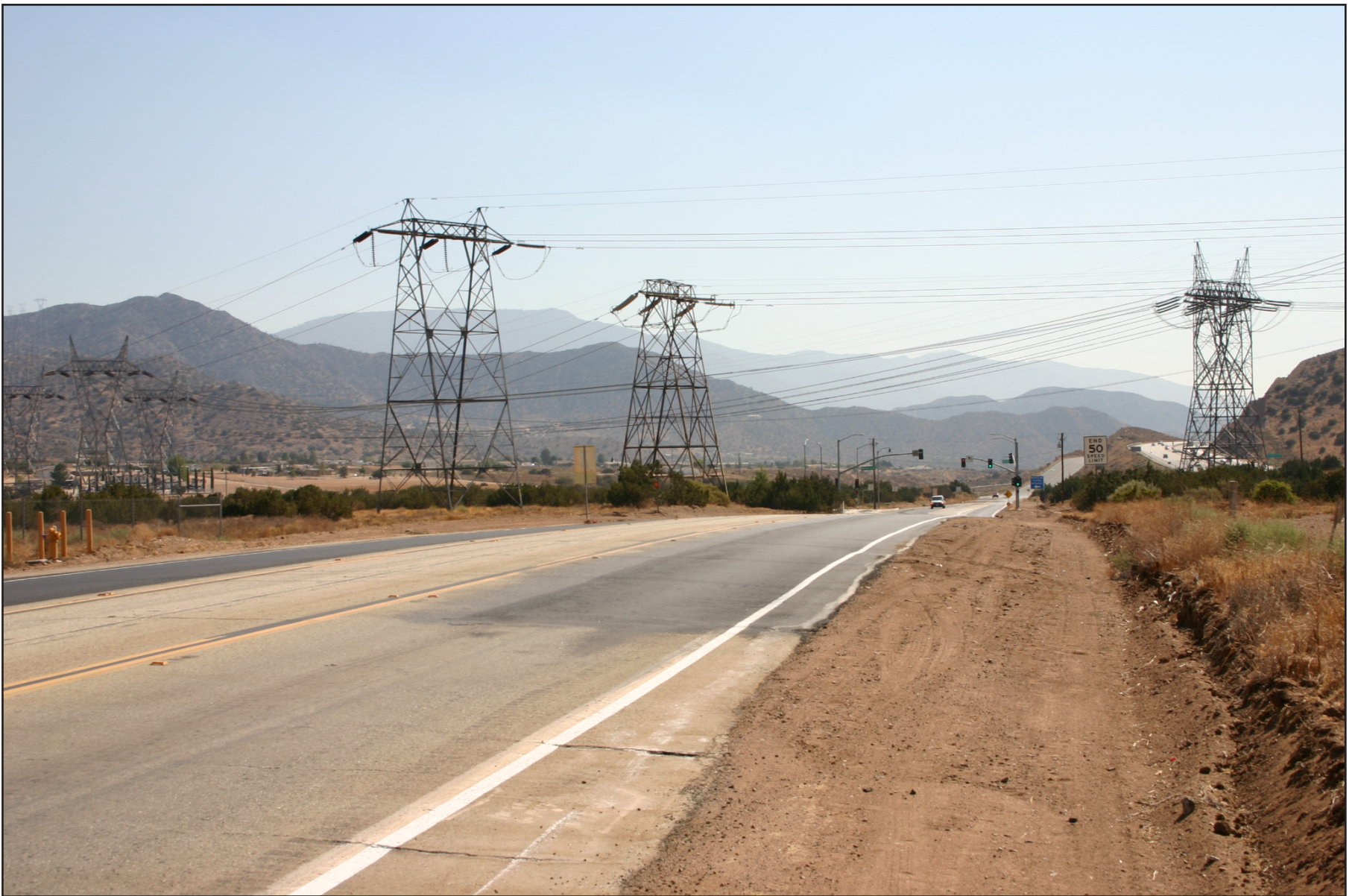
B Addition of new transmission line as seen from KVA Seg 2-3 .
